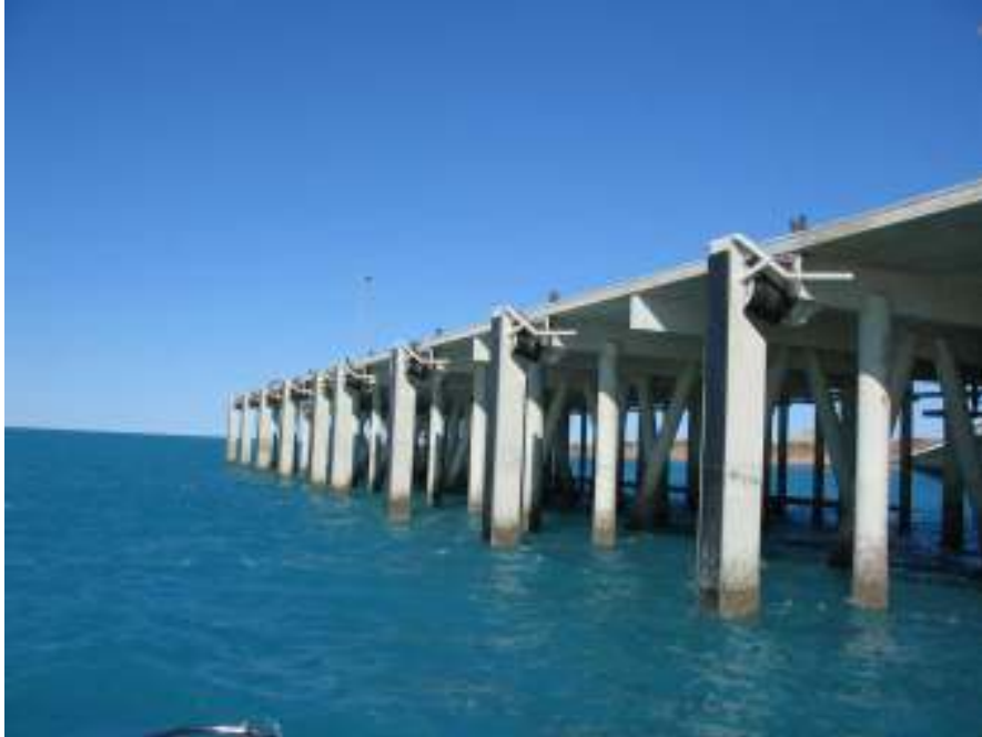
Photograph 1 – Berth 6 viewed from NNE
