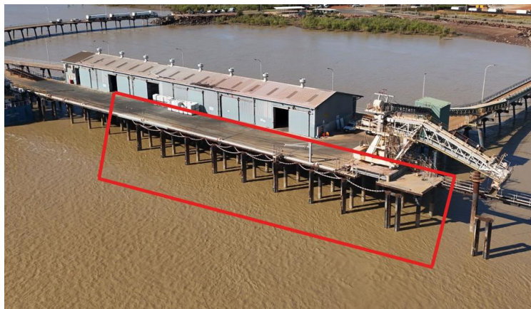
Image showing area of maintenance and repairs
