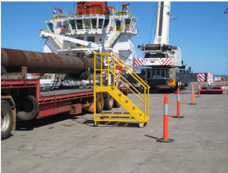
Photo 2: Trailer access and crane/truck work zone
